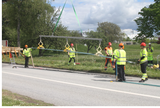
Figure 2.5: Installation of the elevated design.
