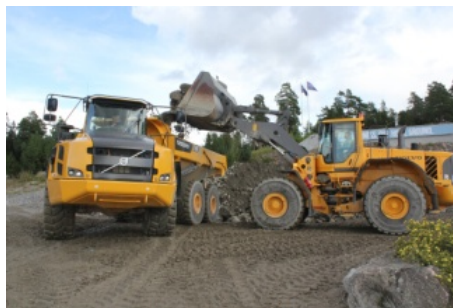
Fig. 2.3 Measurement setup for the “short loading cycle rock”.
