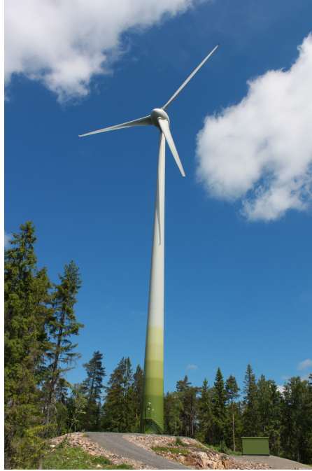
Figure 5.2: Field test wind turbine of type Enercon E-53 with a rated capacity of 800kW and a reactive power capability of \pm 410 kvar.
