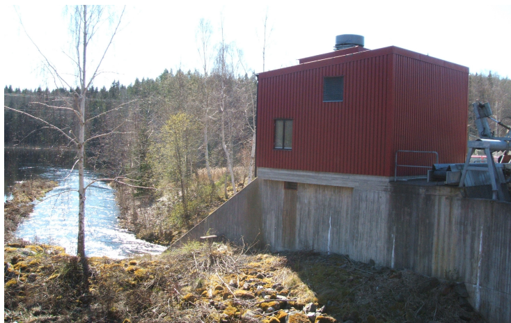
Figure 8.1 Forsa hydro power station with semi-Kaplan turbine and induction generator.
