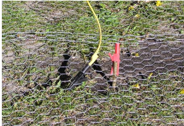
Figure 2.13. The chicken net and the brass bar are electrically connected, and the conductor that can be seen comes from the measurement equipment.
