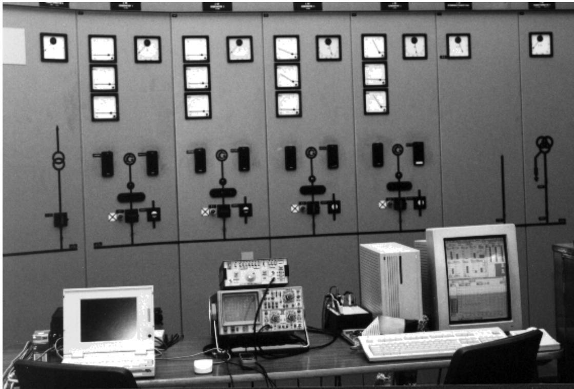
Fig. 6.8 Instruments and computers for control, monitoring and data logging.
