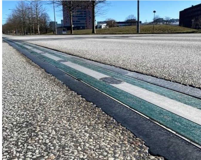
Figure 1. One of the test sites of conductive ERS on public roads in Sweden [11].
