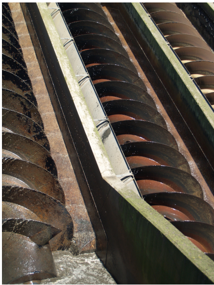
Figure 6.1 Screw pumps
