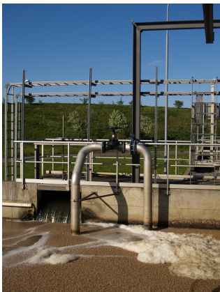
Figure 8.9 Denitrification with suspended carriers
