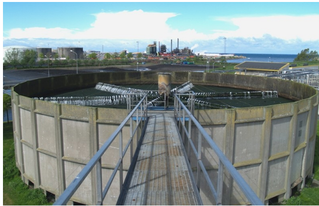
Figure 3.3 Trickling filters
