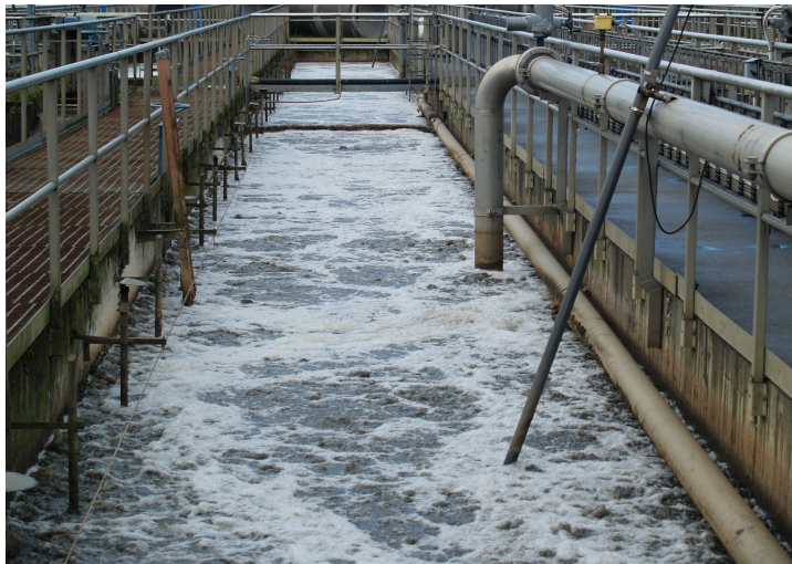
Figure 3.2 Activated sludge process
