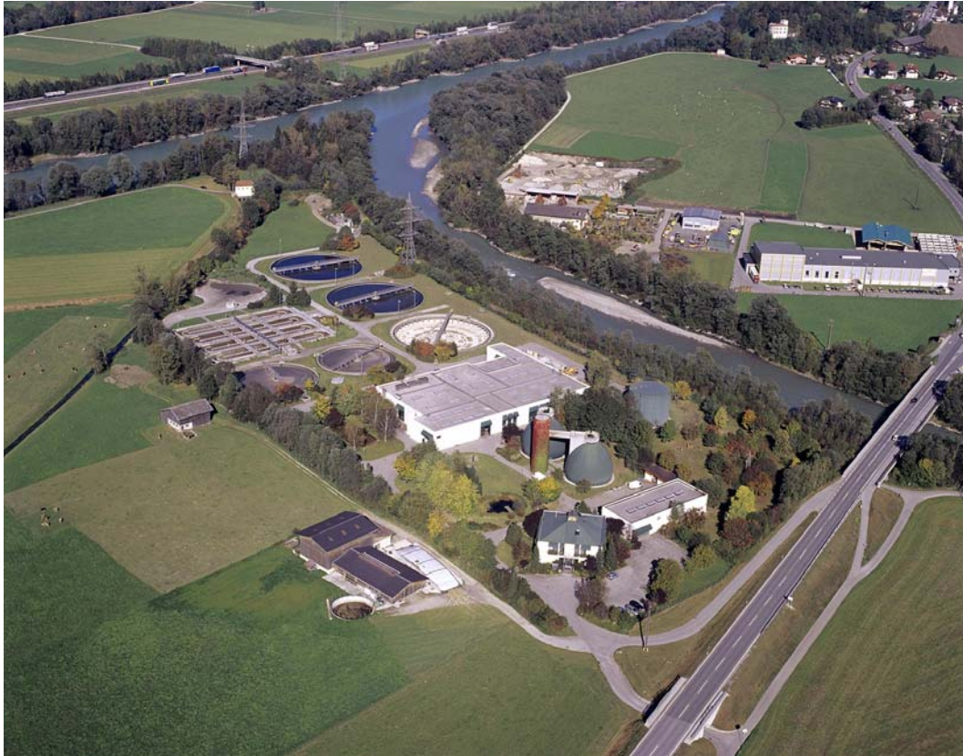
Picture taken in October 1996 ( http://www.aiz.at/klaeranlage.htm ).
